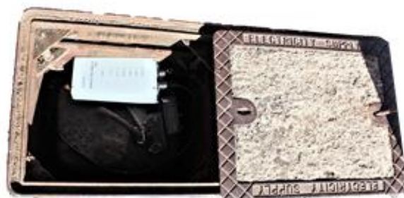
Figure 6.11b: T-P23 laid on top of the link-box bell housing
