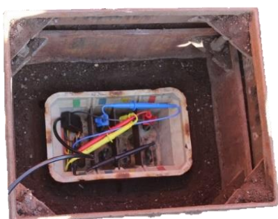
Figure 6.11a: T-P23 connections in the utility link box using clip connectors
