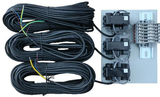
Figure 4.17 CT mounting plate
